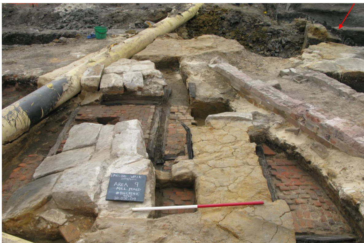
Figure 3.5.52: View of timber and brick floor structure 9241 from the south. It was truncated by a modern service pipe and brick-built culvert, and later sandstone structure 9240 was built over it. Photo taken looking north, the mill pond is located just to the right (arrow). Scale 1m.
