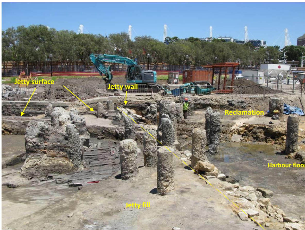
Figure 3.5.11: View of the jetty wall remains from the shore with remains of the jetty in-fill and surfacing. The timber slipway was revealed below the jetty fill. The harbour floor is to the right with reclamation (Phase 5) overlying. View to west. Scale 1m.
