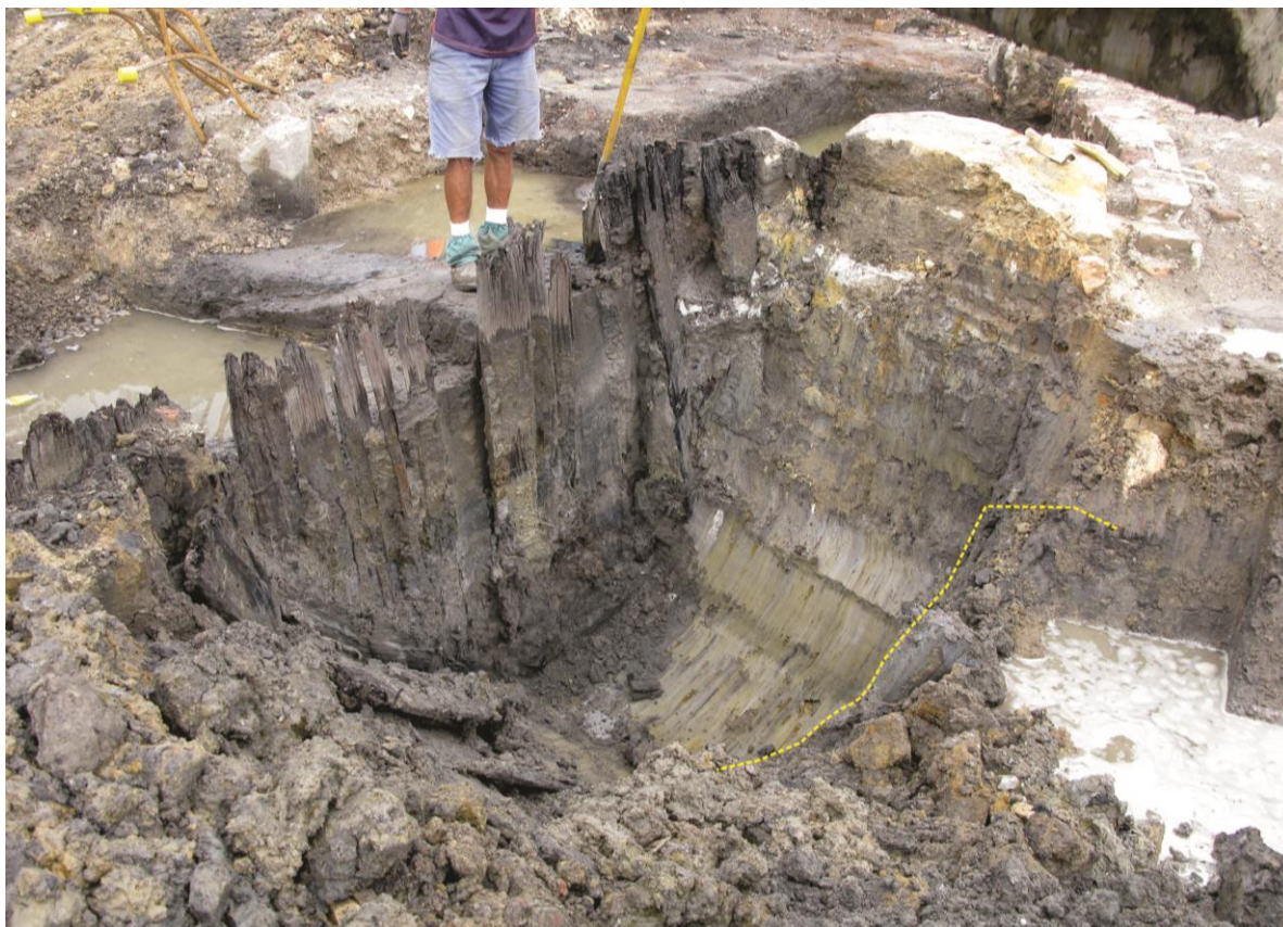
Figure 3.5.44: Machine-excavated test pit at the eastern end of TT69 to investigate the construction of the mill pond. Outside the timber planks forming the mill pond revetment wall was a clay-lined cut, indicated by the dashed yellow line. View to southeast.
