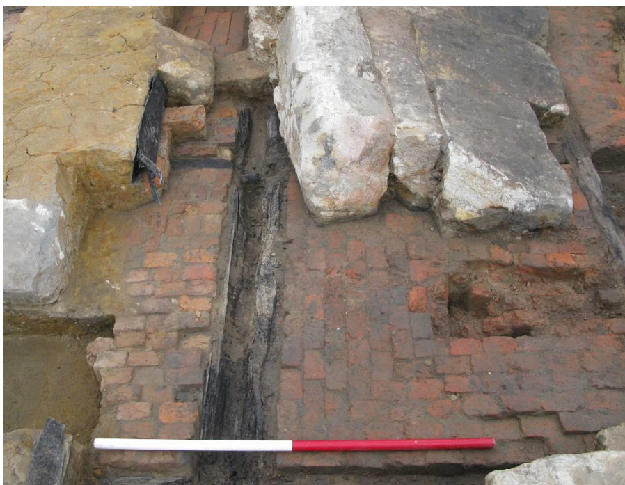
Figure 3.5.54: Detail of the sandstock brick surface inlaid within the timber frame. These were tightly set and placed on their ends with 'mud mortar' filling the gaps. Scale 1m.
