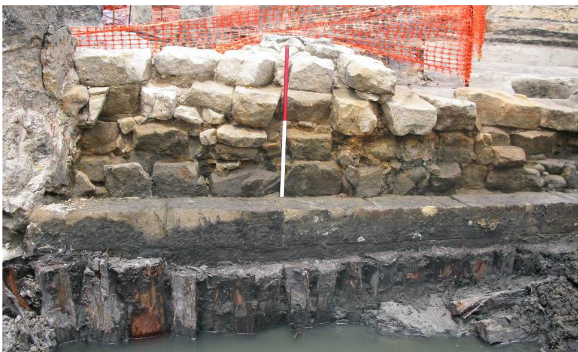
Figure 3.5.14: View of the harbour-side of the jetty wall with the top of the timber formwork exposed. The oyster shells adhering to the stone just above the top of the formwork indicate that the high tide water levels rose to cover the formwork. View to southeast. Scale 1m.
