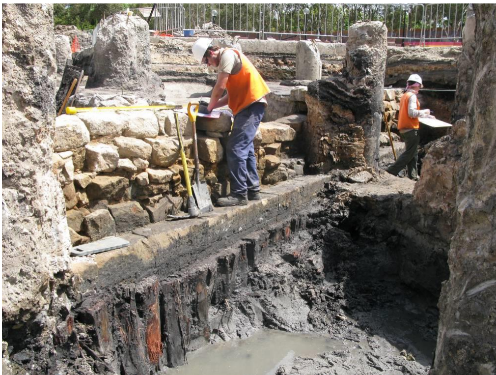
Figure 3.5.23: Recording the jetty remains. The jetty wall was solid sandstone with wooden timber formwork along the harbour side. Grey coarse sands formed the deposits on the harbour-side of the wall. This photo also illustrates the deepening wall courses further into the harbour zone. View to west.
