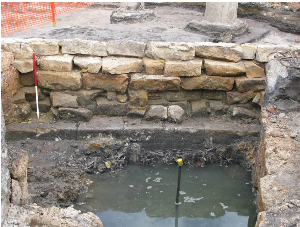
Figure 3.5.21: The jetty wall consisted of ashlar blocks on the harbour face. These were robbed-out before the wall was covered by the reclamation fills in the 1830s. On the internal side of the wall were large rough-cut sandstone blocks. View to the south. Scale 1m.
