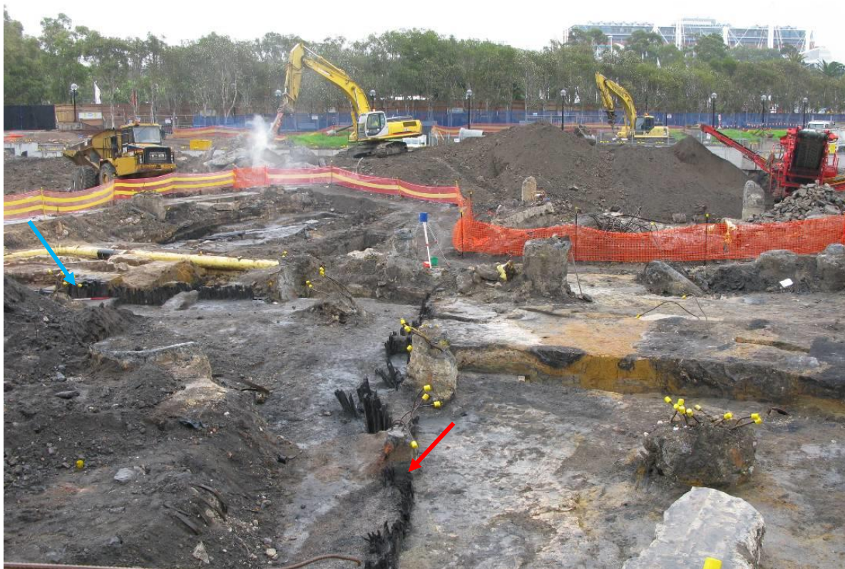
Figure 3.5.39: The timbers formed a revetment on the northwest corner of the mill pond, the red arrow indicates the north wall and the blue the west wall. View to west. Scale 1m.
