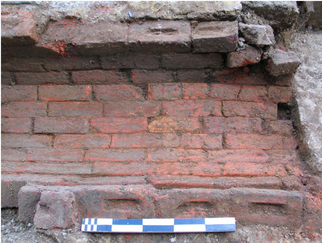
Figure 3.38: Remains of the brick drain (context 7636) that ran along the southern boundary of Lot 2. Scale 500mm.
