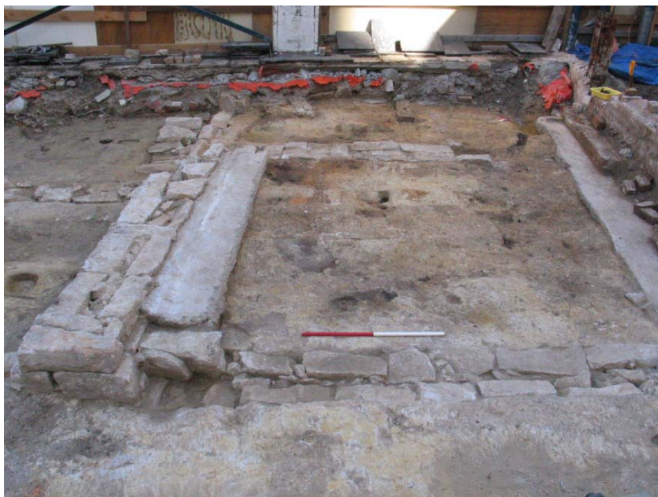
Figure 3.58: The rear room of the structure at No.712 George Street. Concrete has been added to the southern wall and the northern wall has been replaced by a later footing. The internal space showed no evidence of flooring or occupation debris. The partially exposed remains of the front room can be seen beyond. View to the west. Scale 1m.
