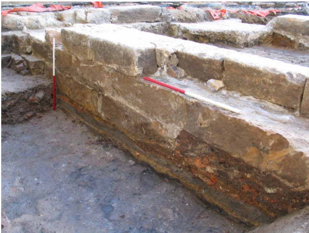
Figure 3.43: Large and well-cut sandstone blocks used in the foundation for the Mercantile Bank. View to the northwest. Scale 1m.
