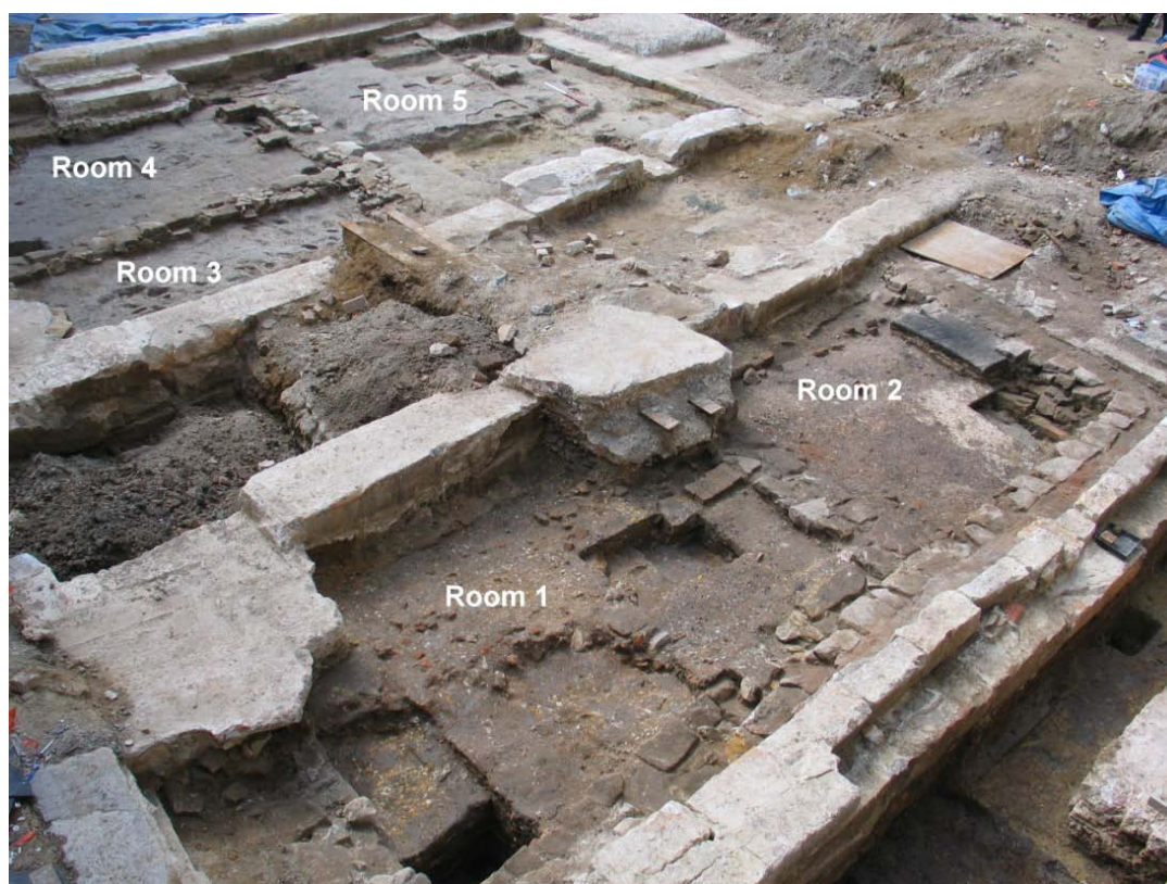
Figure 3.30: The remains of the footings of the Woolpack Inn, showing extensive twentieth-century disturbance in the centre. The sandstone rubble footing is here overshadowed by the much larger concrete and sandstone footing of the later Mercantile Bank. View to the northeast.
