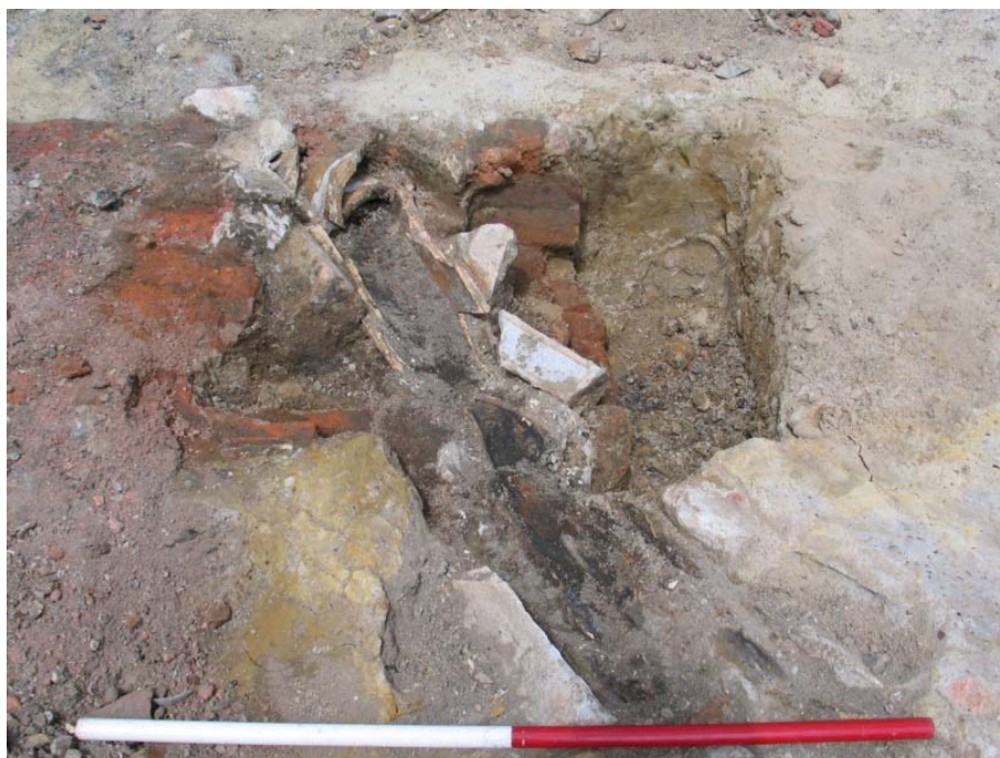
Figure 3.45: The damaged drain in the yard at the rear of the bank building. View to the north. Scale 1m.
