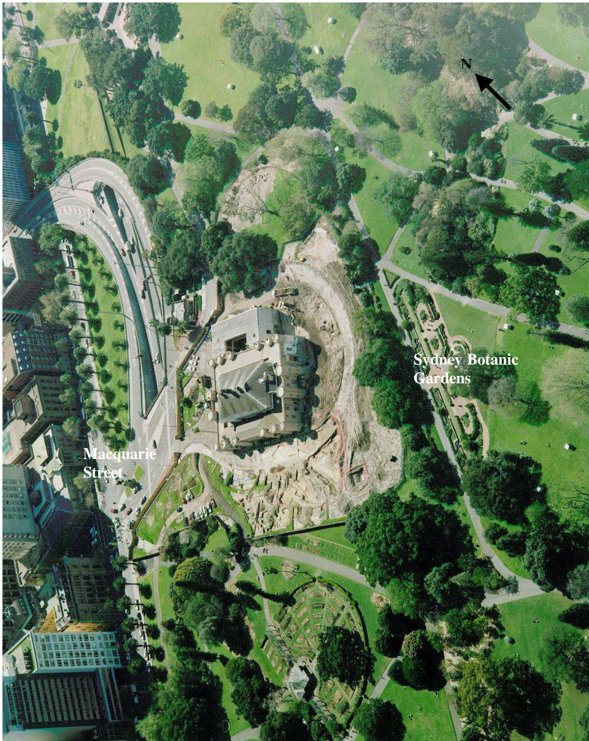
Photo 3.1: Aerial photograph of the Conservatorium site showing Macquarie Street and the Royal Botanic Gardens, 15 September 1998. The main archaeological work was on the southern side of the building. Note that the 1960s building on the northern side has not yet been demolished. Skycam Australia.
